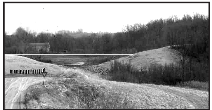
Photograph of dam breach from downstream. White line shows former dam crest, and arrow shows center of breach.
