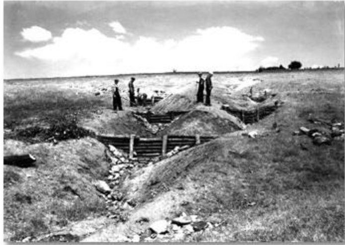
Figure 2 During the 1930s Civilian Conservation Corps crews, such as the one pictured here, worked throughout Ohio to remedy serious erosion problems. This crew works on field erosion barriers at Mohican Forest in preparation for tree planting.
